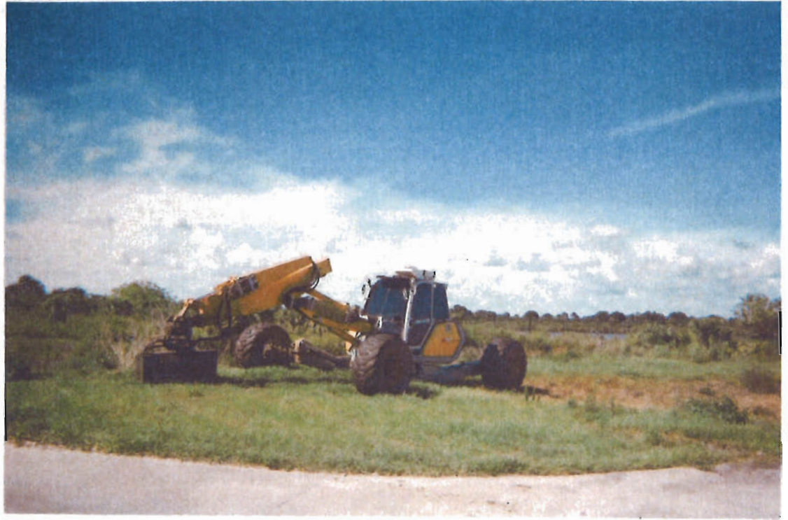
Central Charlotte Drainage District Charlotte County doing canal maintenance
